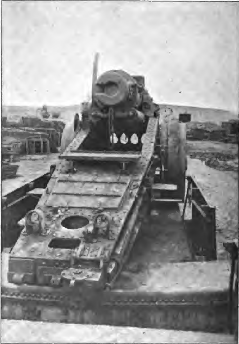
TRAVERSING GEAR OF THE 170 MM. GERMAN GUN MOUNT.
